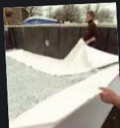
Fitting of the liner
